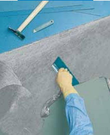
Spreading Ultrabond Eco V4 Conductive
